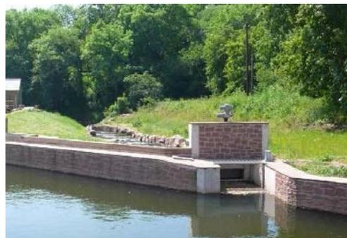
He also introduced a number of detailed designs including the fish pass channel and the inlet structure, which incorporates a penstock and an advanced electronic fish counter. His design incorporates a series of low-head blockstone weirs (figure 2, below) which divide the 3 metre head drop over the weir into a series of navigable 0.3m increments in water level.
