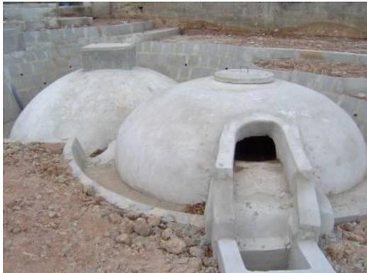
Figure 2: Photo of a fixed dome biodigester before covering with earth.
